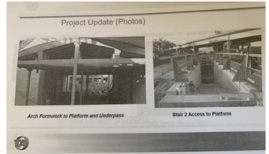
Underpass & Platform Access
