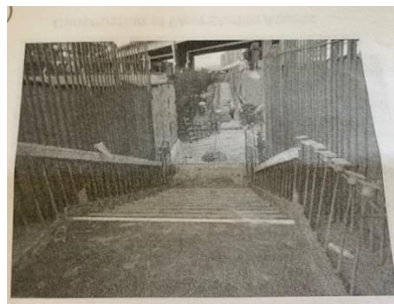
Construction of Ramp 2 Access to Platform
